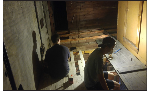
Graduate Brother Keith Downes '91 and Brother Jonathan Robinson '19 replacing old flooring.
