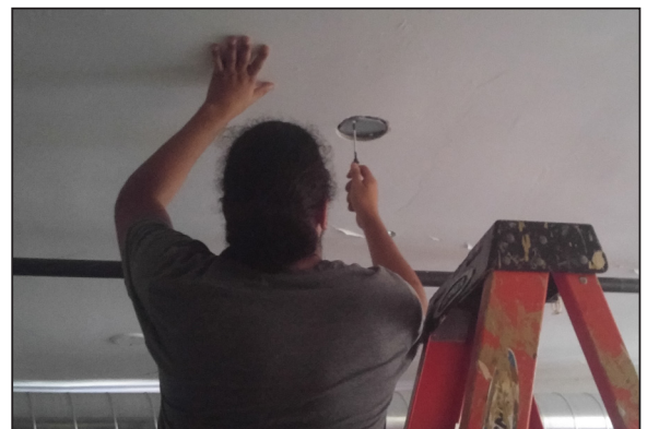
Brother Deslandes '18 fixing lighting on the first floor.
