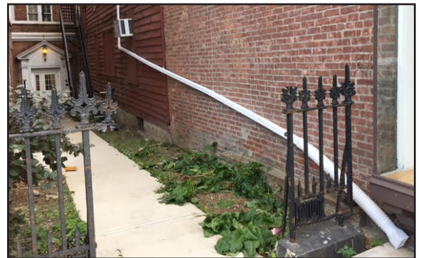
The newly installed gutter.
